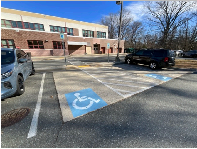
OVERVIEW OF ACCESSIBLE PARKING AREA
