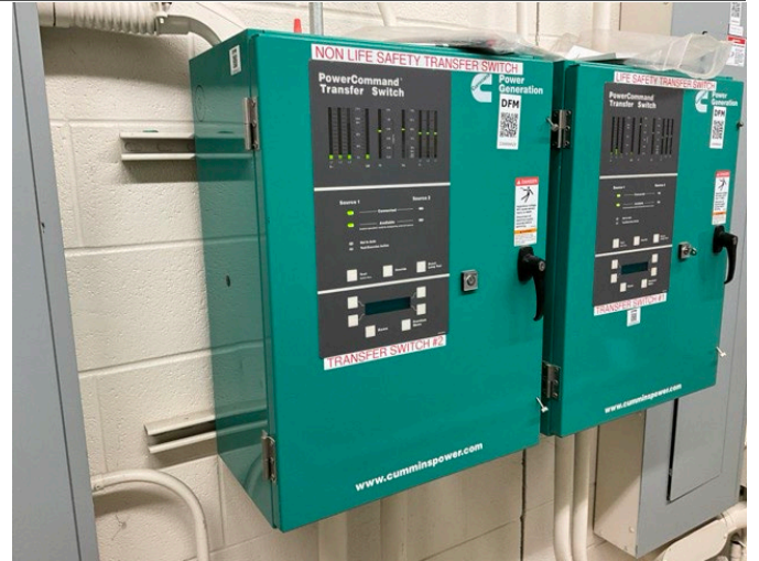
20 - AUTOMATIC TRANSFER SWITCHES
