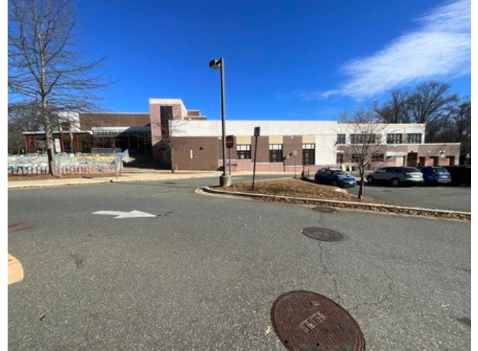
26 - SECOND PARKING LOT VIEW
